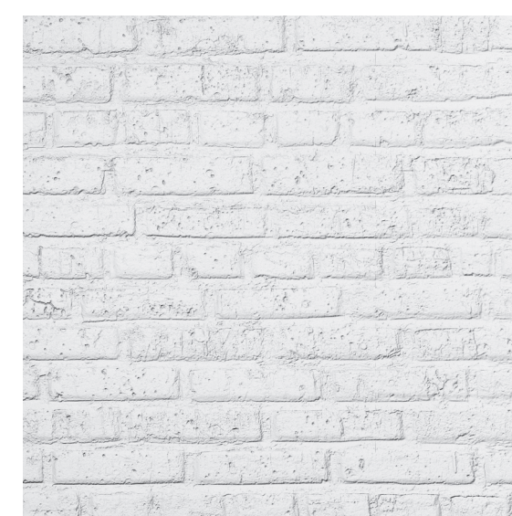
EXISTING WHITE BRICK
